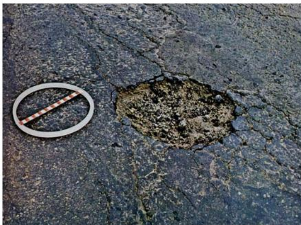
Figura 20: Painela/ buraco
